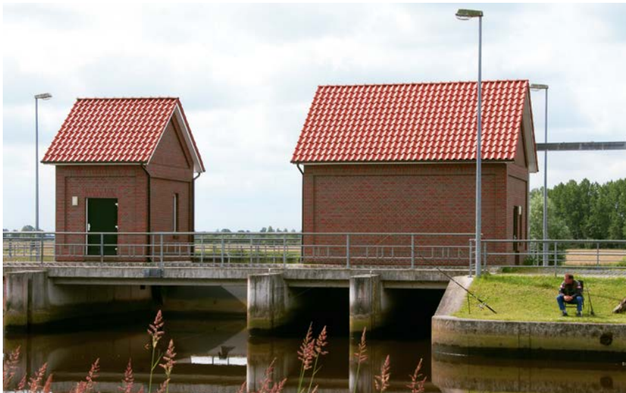
Pumpenhäuser in Detern Bockhorner Bunt 04 Glatt OF
